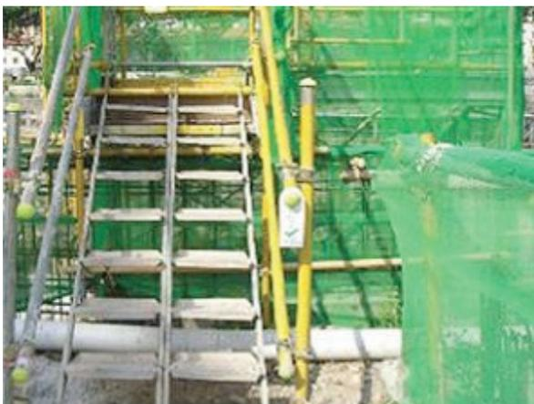
Figure 3 Proper means of access to scaffolds
