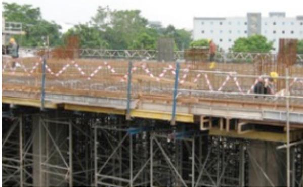
Figure 7 Barricades for open sides, marked with tape for visibility
