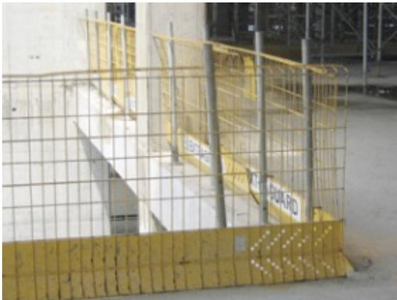
Figure 1 Perimeter guard-railing
