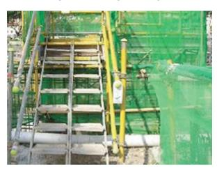
Figure 3 Proper means of access to scaffolds
