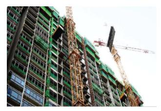
Figure 5 Example of netting for high rise construction
