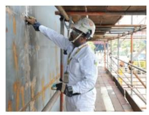
Figure 6 Working platform with guardrails and toe boards installed
