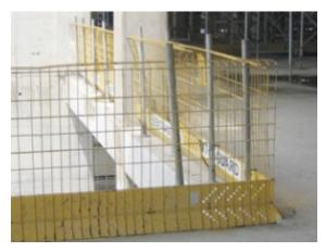
Figure 1 Perimeter guard-railing
