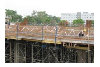
Figure 7 Barricades for open sides, marked with tape for visibility
