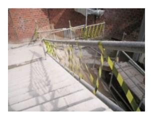
Figure 2 Handrails at open edges of stairway
