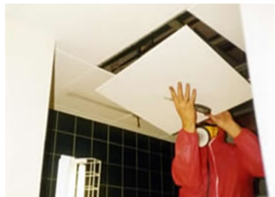
Careful handling of an AIB ceiling tile during removal
