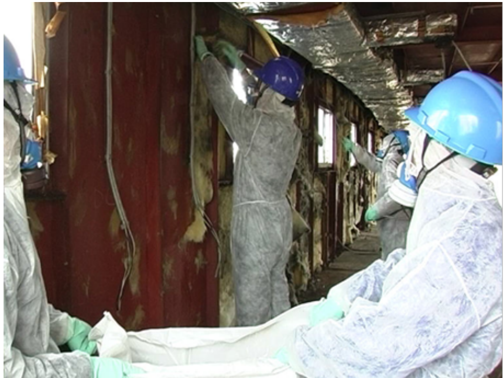
Asbestos workers wearing Personal Protective Equipment
