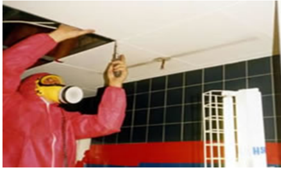
Unscrewing of an AIB ceiling tile
