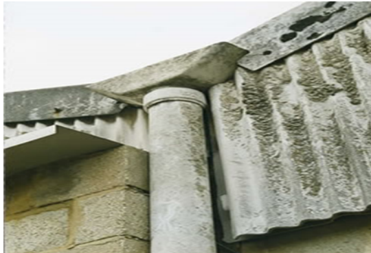
Asbestos cement downpipe, hopper and profile sheet
