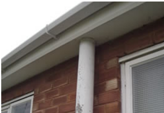
Asbestos cement drainage pipe (down pipe)
