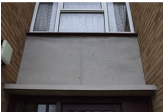
Asbestos cement external building panel
