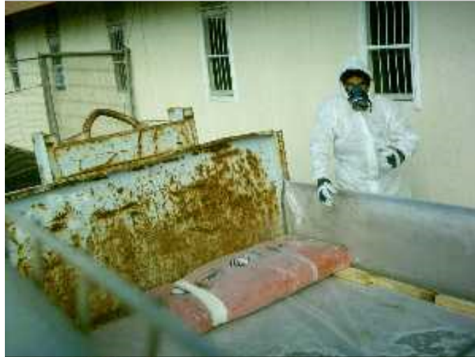
Asbestos bagged up and ready for disposal
