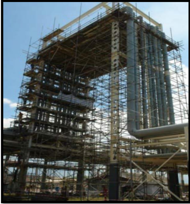
Figure 4 – Bird Cage Scaffold using Tubes and Clamps
