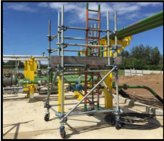
Figure 2 - Mobile Scaffold using Tubes and Clamps
