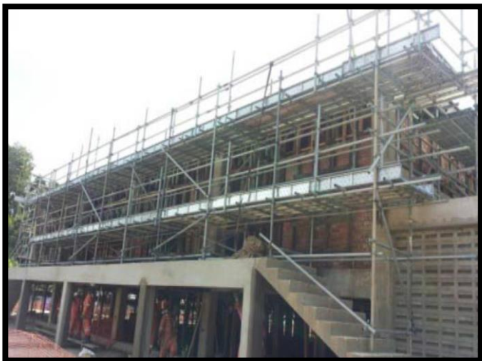
Figure 3 (b) – Independent Scaffold using Tubes and Clamps for Building Construction
