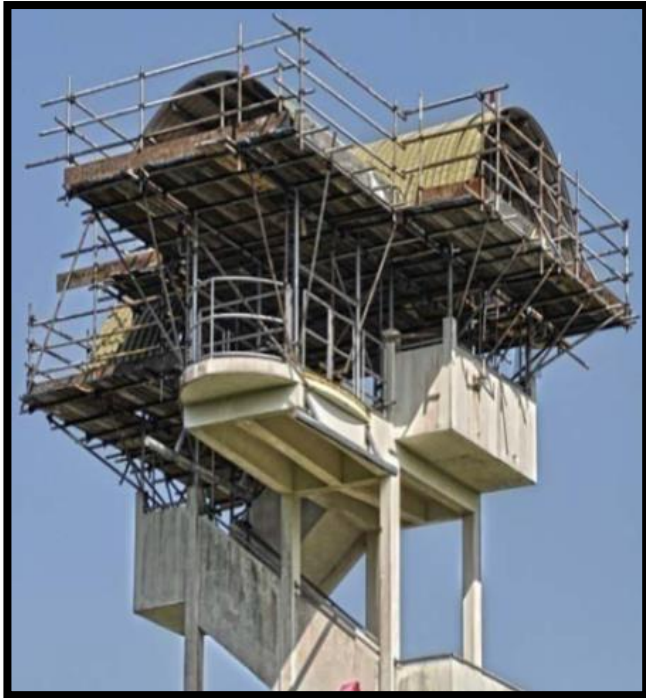
Figure 7 – Cantilever Scaffold using Tubes and Clamps
