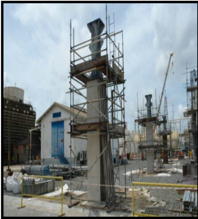
Figure 1 (a) - Static Tower Scaffold using Tubes and Clamp for Pipe Support
