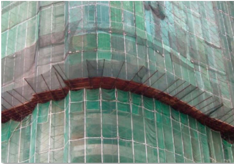
Figure 8: Use of safety net around scaffold
