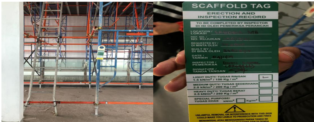
Figure 14.1 Scaffolds have to be certified and tagged as safe before use.
