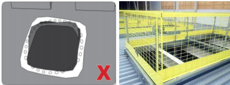
Fig.2 Unsecured openings are a hazard that can lead to serious injury or even death (L), an example of fenced floor opening (R, photo credit: www.safetyrespect.com ).
