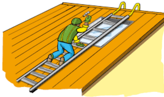
Fig. 6: Illustration of worker using crawling board as protection from sliding off roof ( picture credit: ilo.org )
